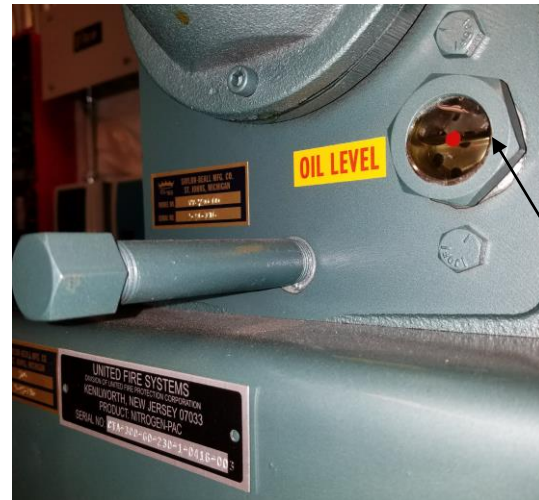
FIGURE 4 – OIL LEVEL SIGHT GLASS
