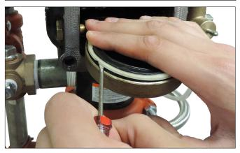
Pry the clapper seal, along with the seal ring, out of the clapper. 6. Inspect the clapper seal. If the clapper seal is torn or worn, replace it with a new, Victaulic-supplied clapper seal. If replacing the clapper seal assembly with a new assembly, skip to step 7.
