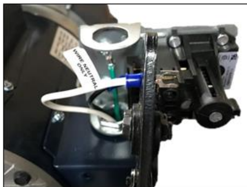
5. Crimp a spade connector onto NEUTRAL wire.
