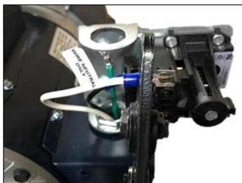
5. Crimp a spade connector onto NEUTRAL wire.
