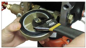
2. Remove the seal assembly bolt/bolt seal from the clapper seal.
