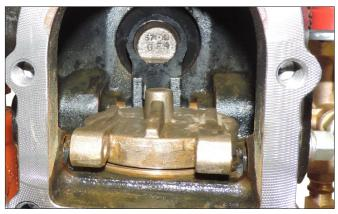
Place the new clapper assembly onto the valve body seat ring. Verify that the holes in the clapper arms align with the holes in the valve body.
