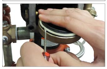
5. Pry the clapper seal, along with the seal ring, out of the clapper. Inspect the clapper seal. If the clapper seal is torn or worn, replace it with a new, Victaulic-supplied clapper seal. If replacing the clapper seal assembly with a new assembly, skip to step 7.
